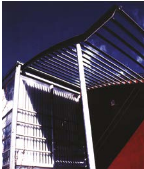
16 | Solar shading in SA1, Swansea
