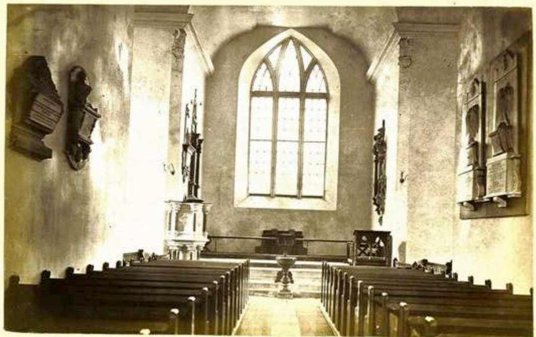
St. Mary's Church - looking east -
