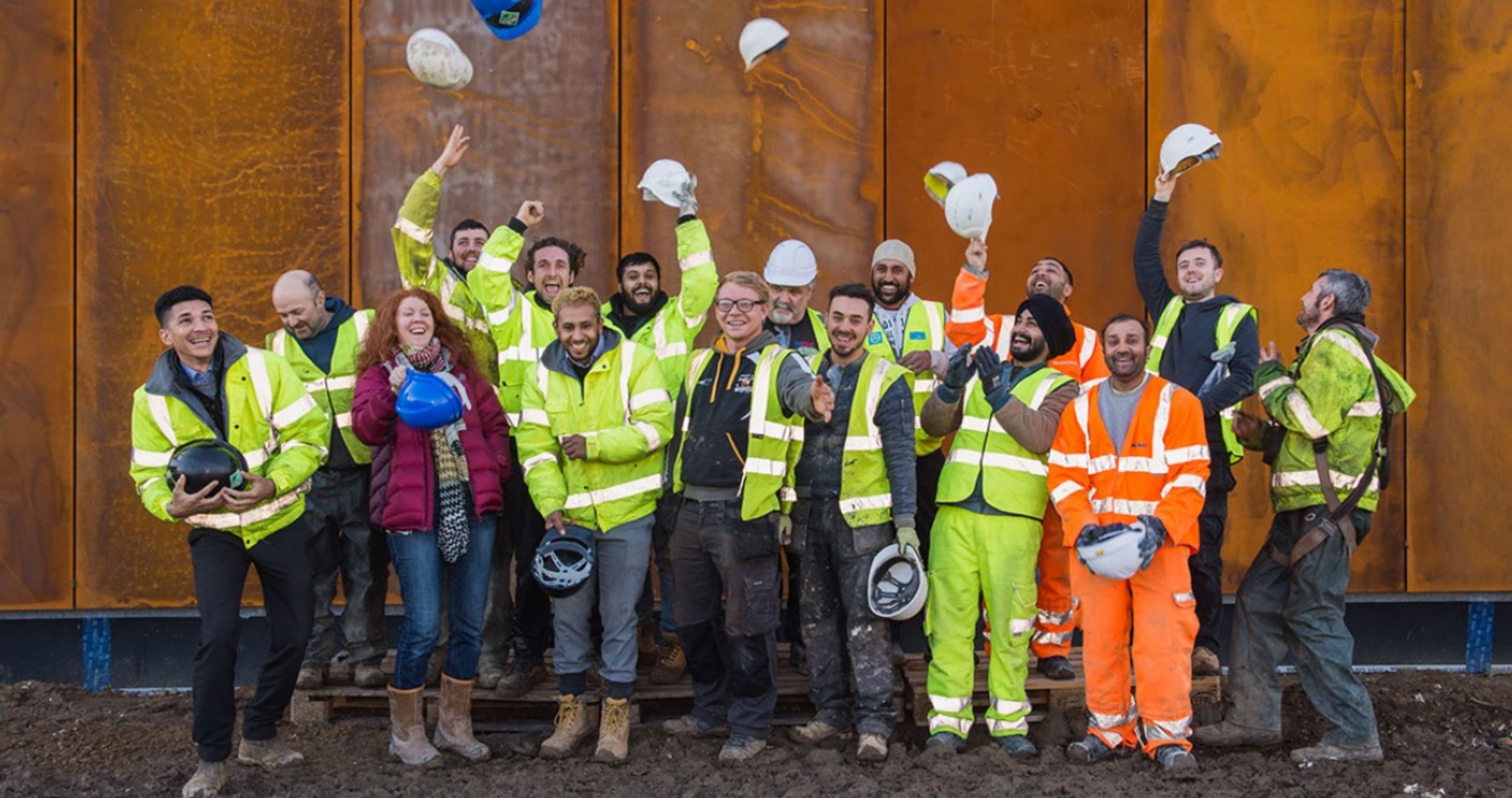
Site team celebrate achieving the world airtightness record on IWM Context: IWM was their very 1 st Passivhaus build and toolbox talks were invaluable
