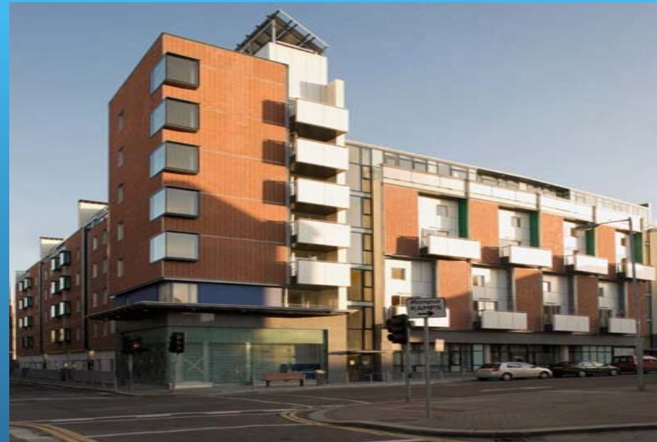
York Street Housing - Dublin
