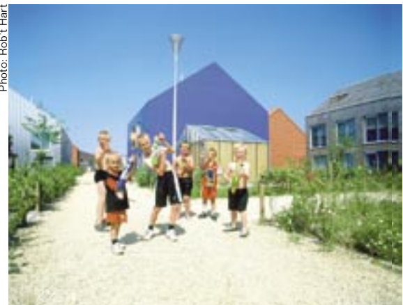
Housing development, Hagen Island, The Netherlands. Architects: Winy Maas, Jacob van Rijs, Nathalie de Vries, MVRDV. Award won: Special Mention European Union Prize for Contemporary Architecture – Mies van der Rohe Award 2003.
