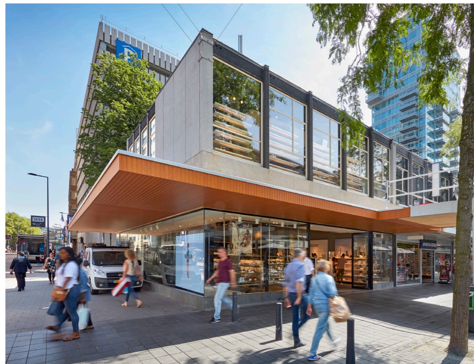
Renovation of the world famous as the first car-free shopping promenade | Lijnbaan, Rotterdam, NL
