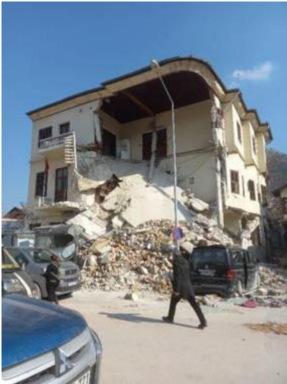
Examples of damages to civil architecture works in the historical city centre of Antakya after the earthquake of 6 February 2023 (Photograph: Assoc. Prof. Dr. Koray Güler)
