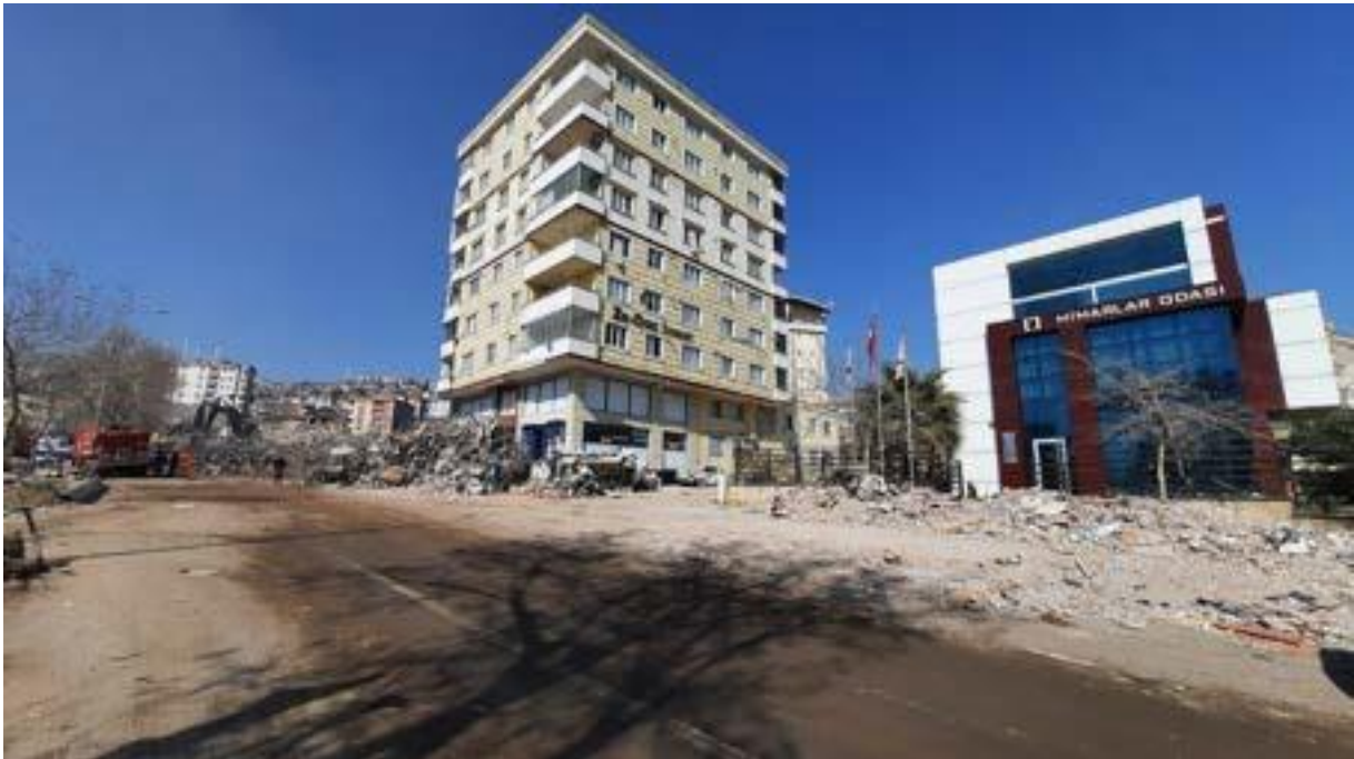
Chamber of Architects Kahramanmaraş Branch Building
