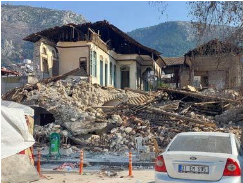
Examples of damages to civil architectural works in the historical city centre of Antakya caused by the earthquake of 6 February 2023
