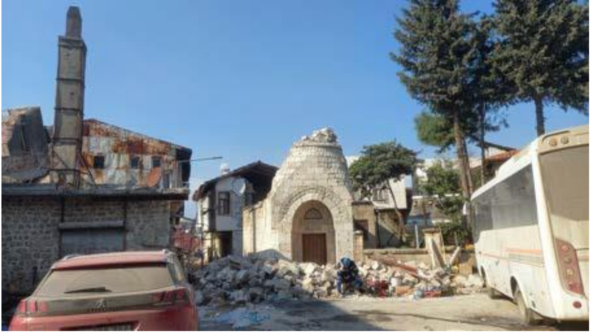
Post-earthquake view of Sarimiye Mosque in Hatay (Photograph: Assoc. Prof. Dr. Koray Güler)
