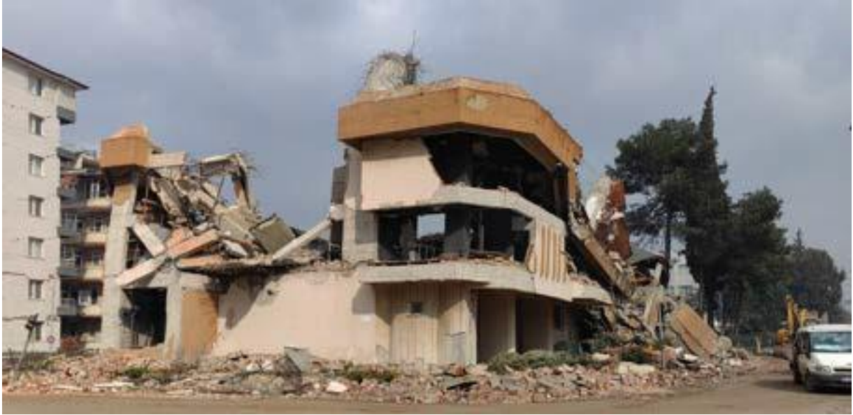
Damage to Hatay Cultural Centre after the earthquake of 20 February 2023
