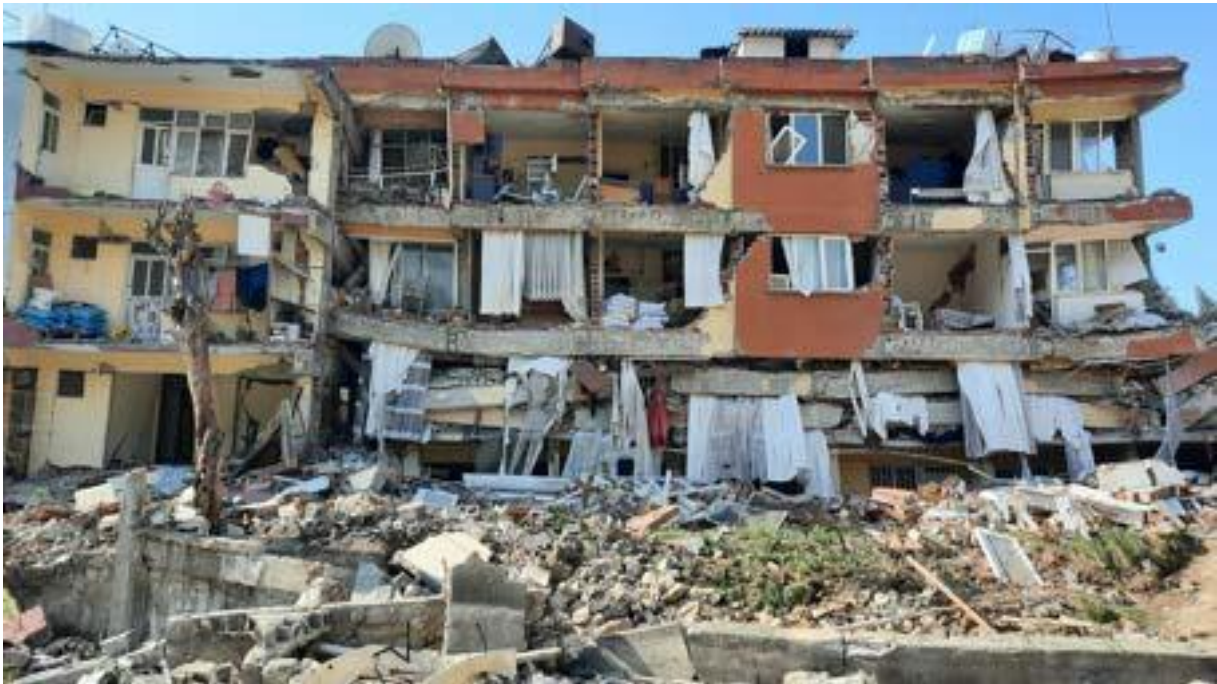
Hatay - heavily damaged and demolished buildings in the city centre
