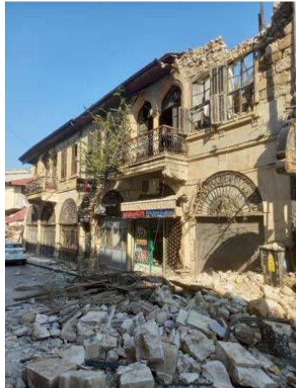
Examples of damages to civil architecture works in the historical city centre of Antakya after the earthquake of 6 February 2023 (Photograph: Assoc. Prof. Dr. Koray Güler)
