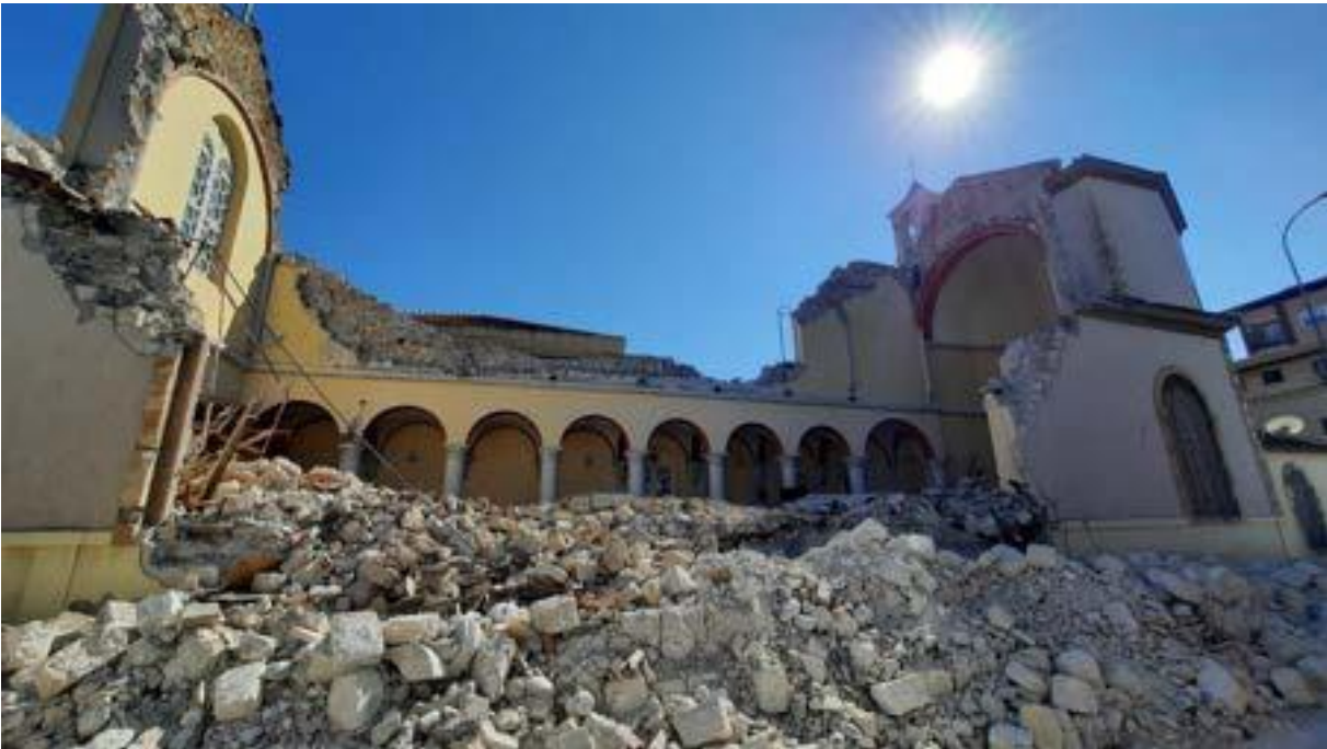
Iskenderun Latin Catholic Church after earthquake damage
