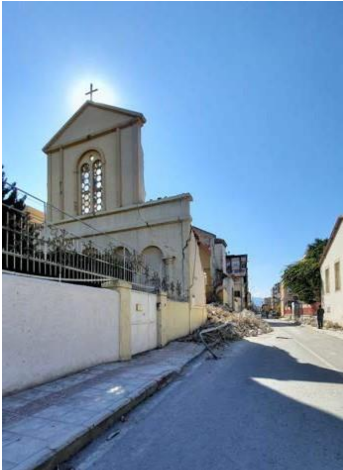
Iskenderun Latin Catholic Church after earthquake damage
