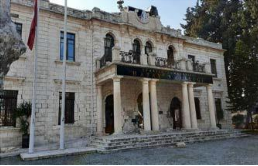
Hatay Government House (Governorship) damaged after the earthquakes of 6 February 2023
