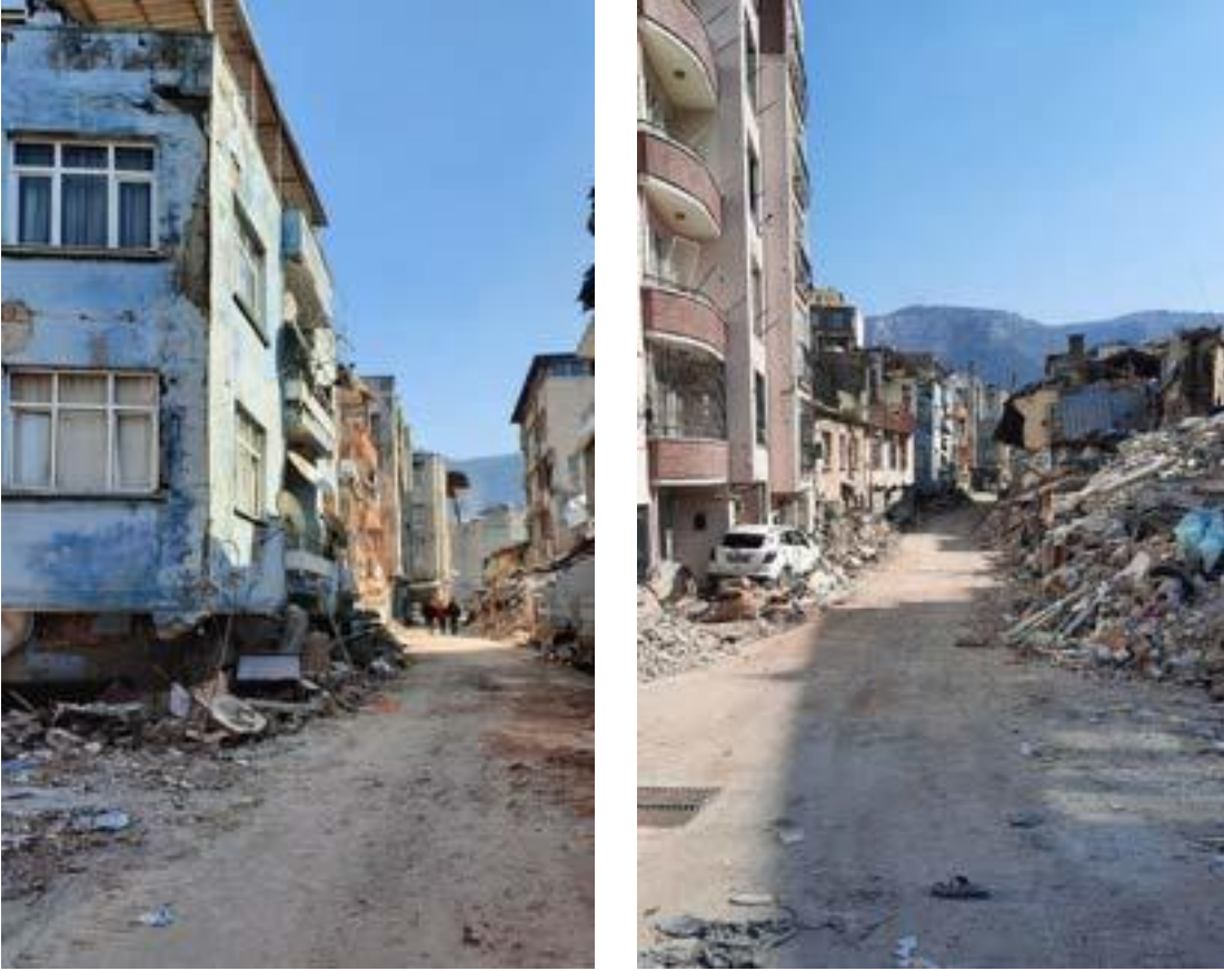
Damage to Hatay city centre after the earthquakes of 6 February 2023
