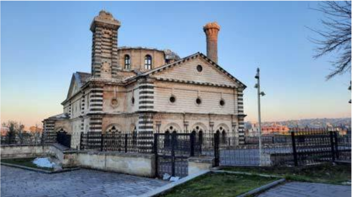
Damages observed in Kurtuluş Mosque after the earthquake
